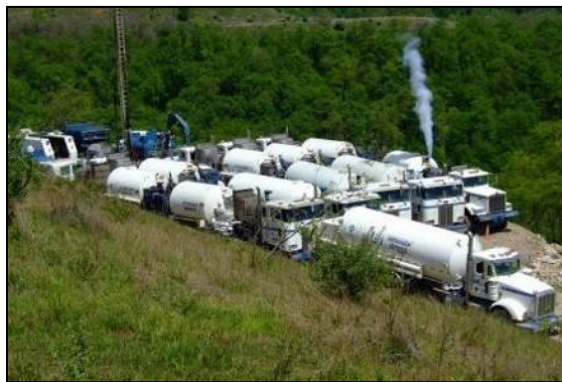
Figure 157 Foam Frac equipment on location
