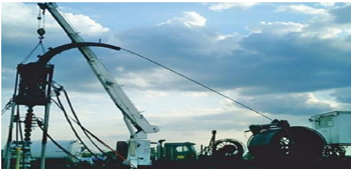
Figure 149 General coiled tubing rig up
