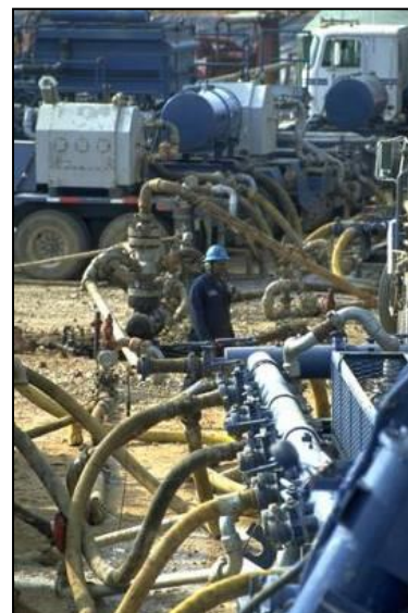
Figure 156 Rig-up Frac pumps to Well Head
