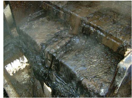
Figure 6 Solids removal at the shale shaker
